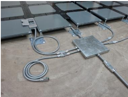
ZoneTeq MWS distributes under low-profile access floor, and under conventional access floor as well.
