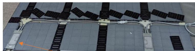
series connection and extension of floor boxes.
