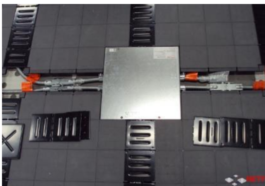
ZoneTeq MWS accommodates Netfloor ECO series low-profile access floors.
